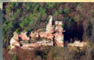
Burgruine/Ruines de château/castle ruins Lützelhaardt/F
